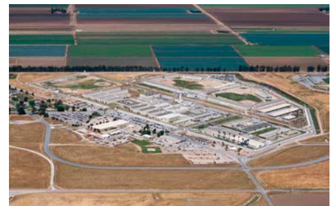
Pitchess Detention Center, New Barracks
