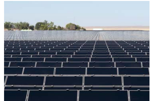
Topaz Solar Farm
