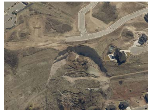
North Salt Lake Landslide
