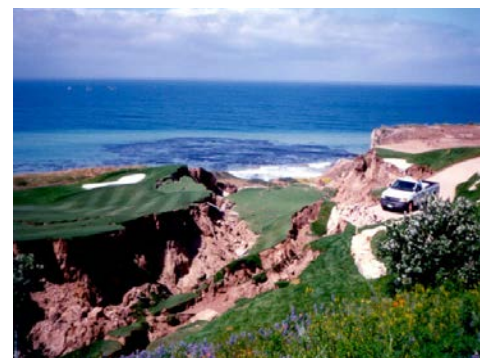
Ocean Trails Landslide
