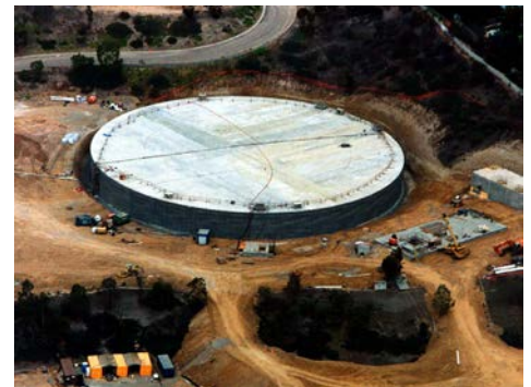
Miramar Storage Tank
