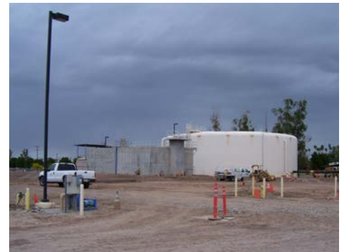
Holtville Water Reservoir
