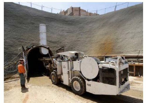
Mission Trails Pipeline Tunnel
