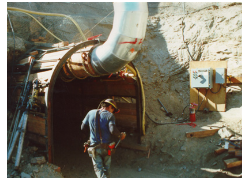
SDCWA Pipeline 2A Tunnel
